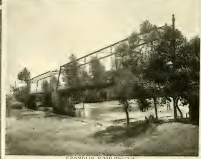
FRANKLIN ROAD BRIDGE
